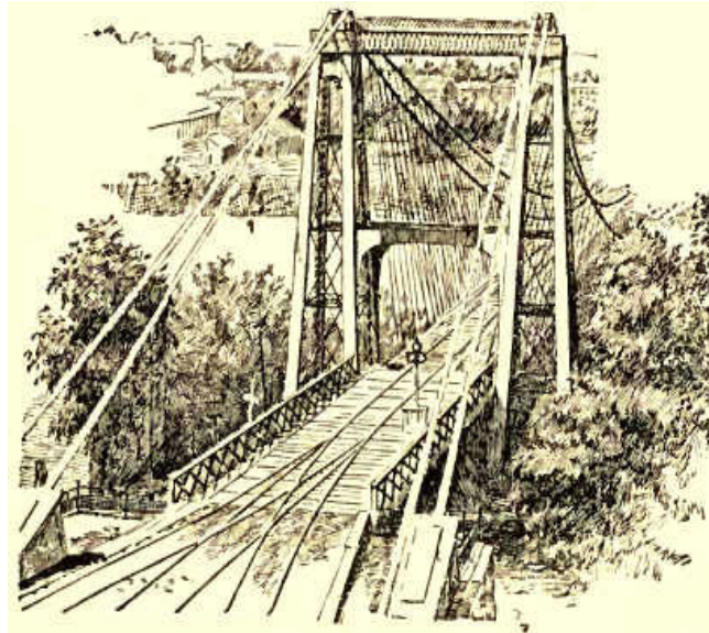
The New Iron Towers of the Niagara Bridge.
